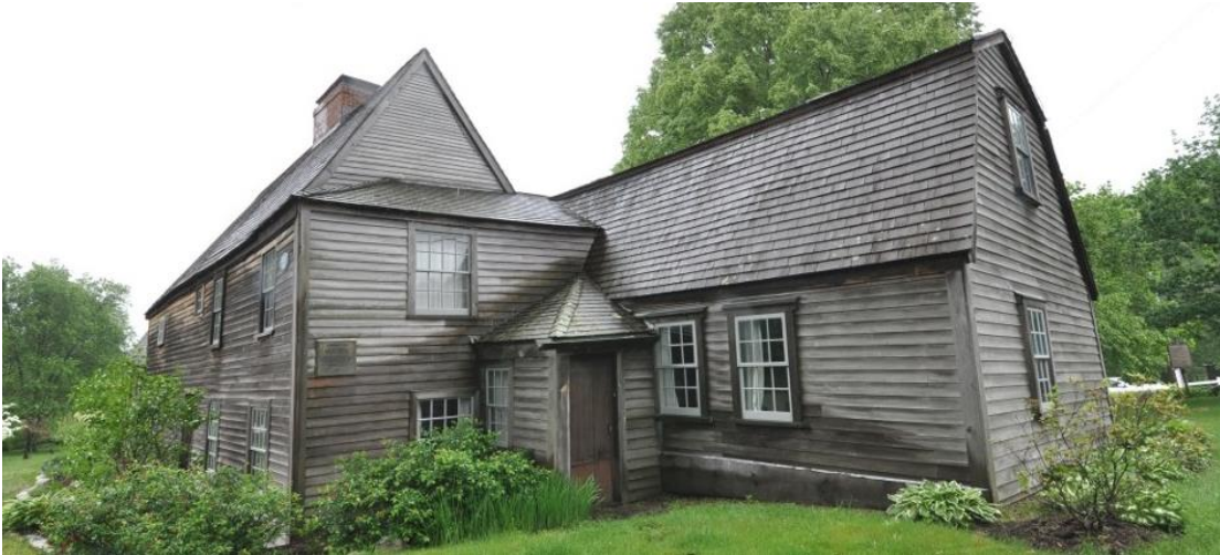
The Jonathan Fairbank Family Home a The oldest part of the house which Jonathan built is on the left.
